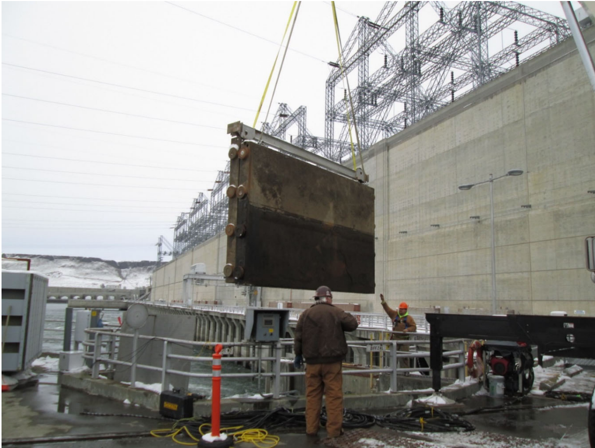
Oregon south entrance weir coming out of the slot.
