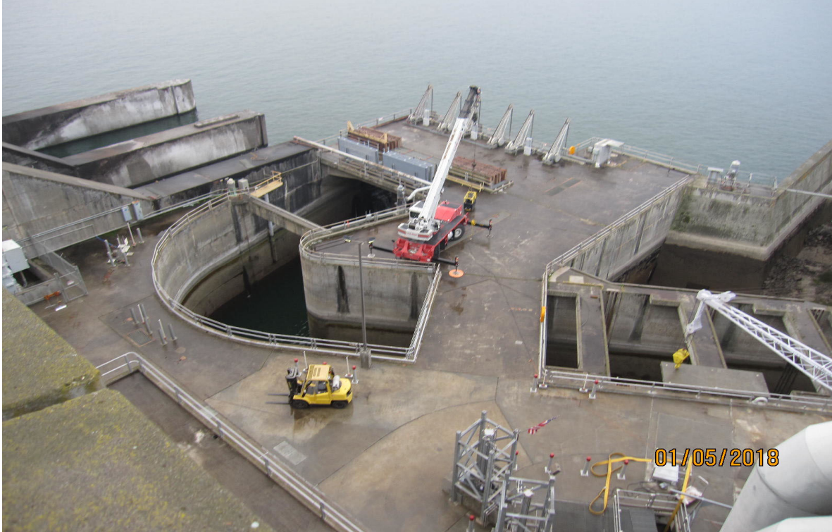
Washington entrance with crane set up to remove weirs.
