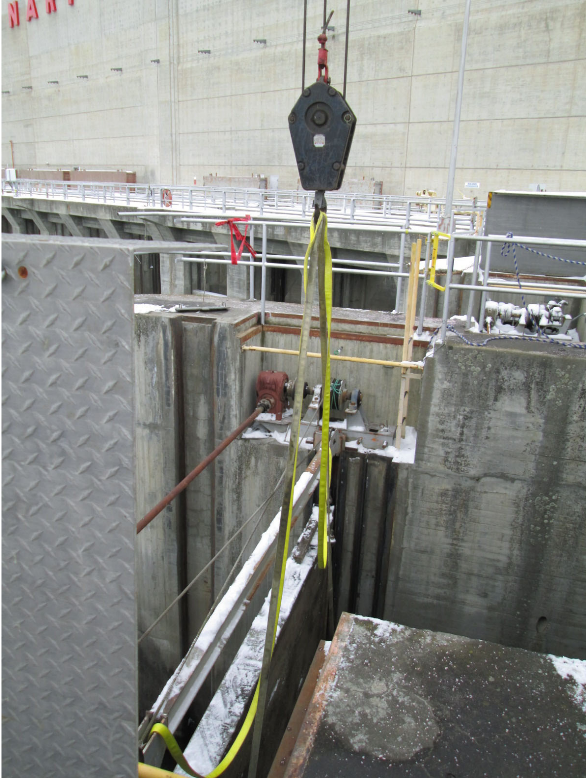
Removing an Oregon south entrance weir.
