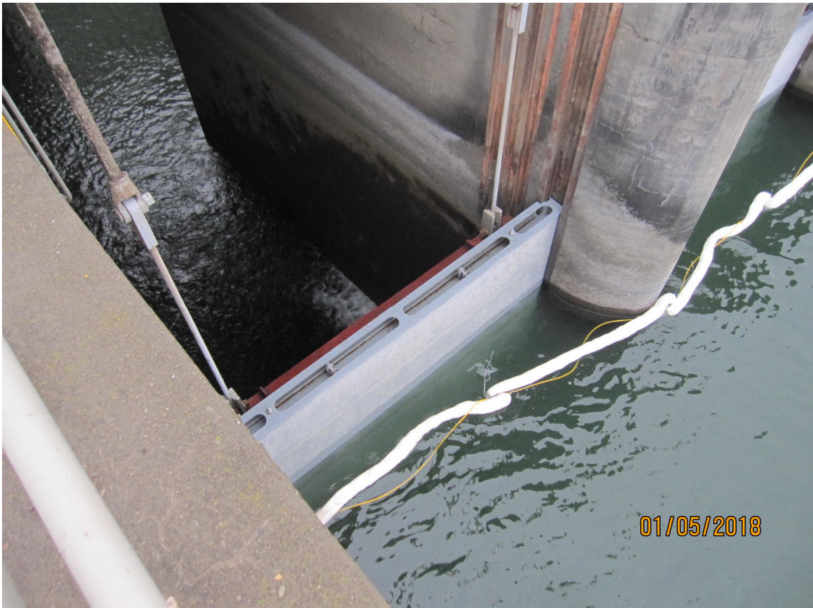
Example of Washington entrance weir with stop logs in place in front of the weir.
