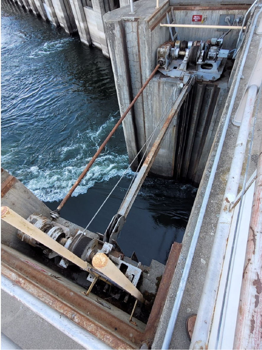
Oregon ladder south entrance weir in the slot.
